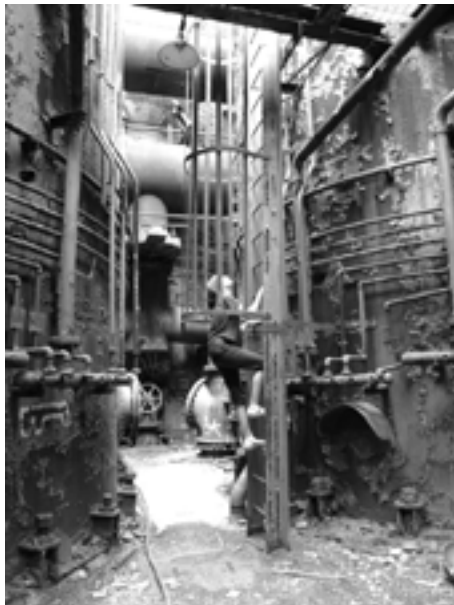
Lara climbing a ladder at the Carrie Blast Furnace site in Rankin, PA.
