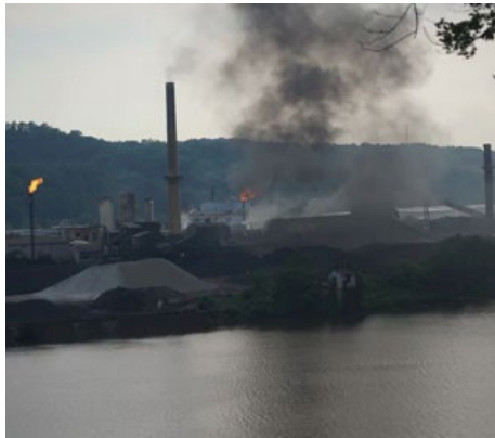
Shenango Coke Plant, June 11, 2015 at 6 PM
